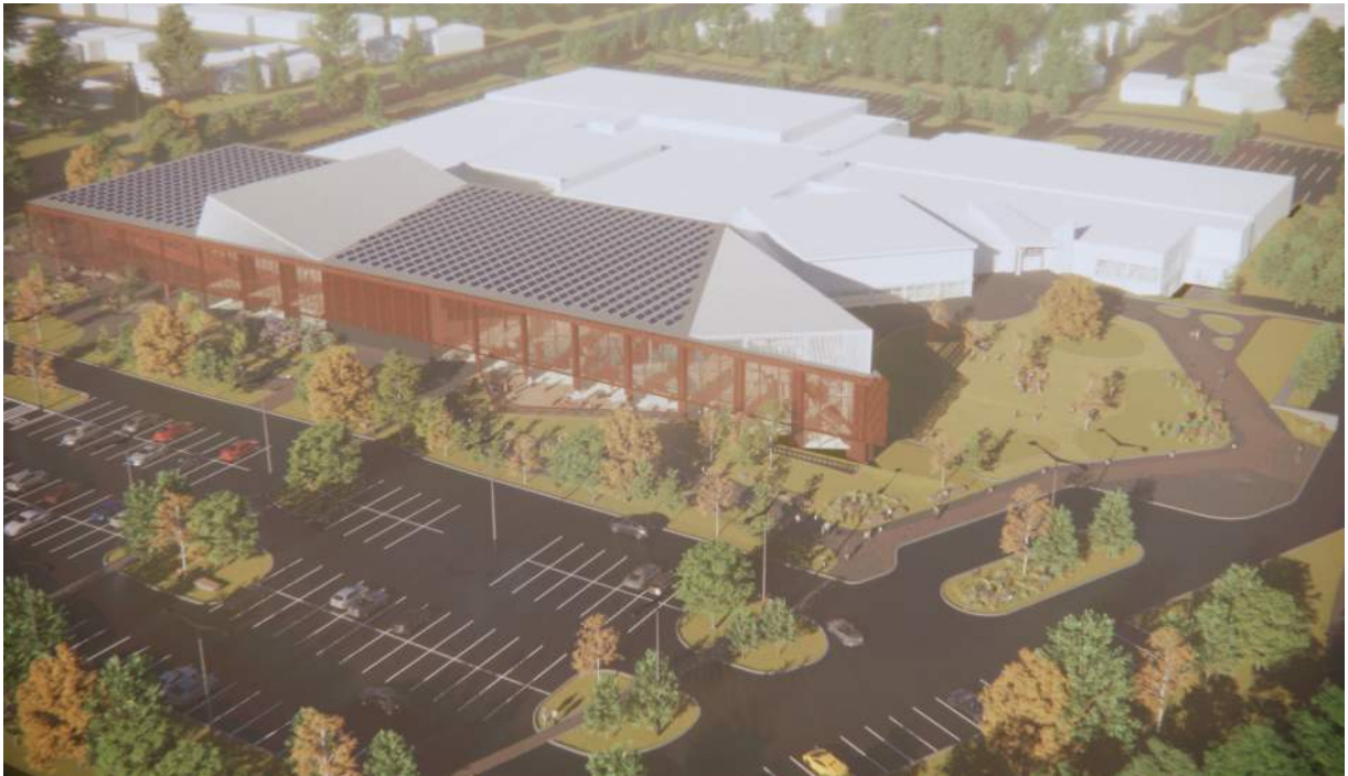
Building Exterior - Southwest Aerial (Phase 1)
