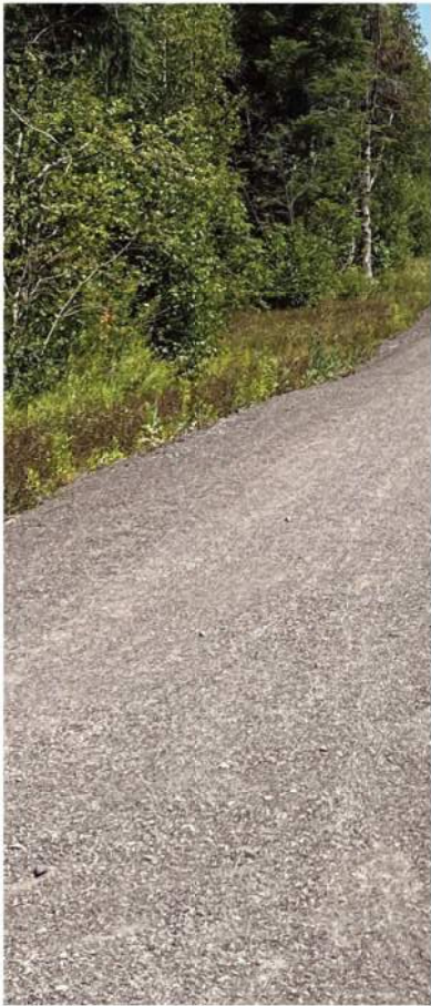
Crusher Dust Paving
