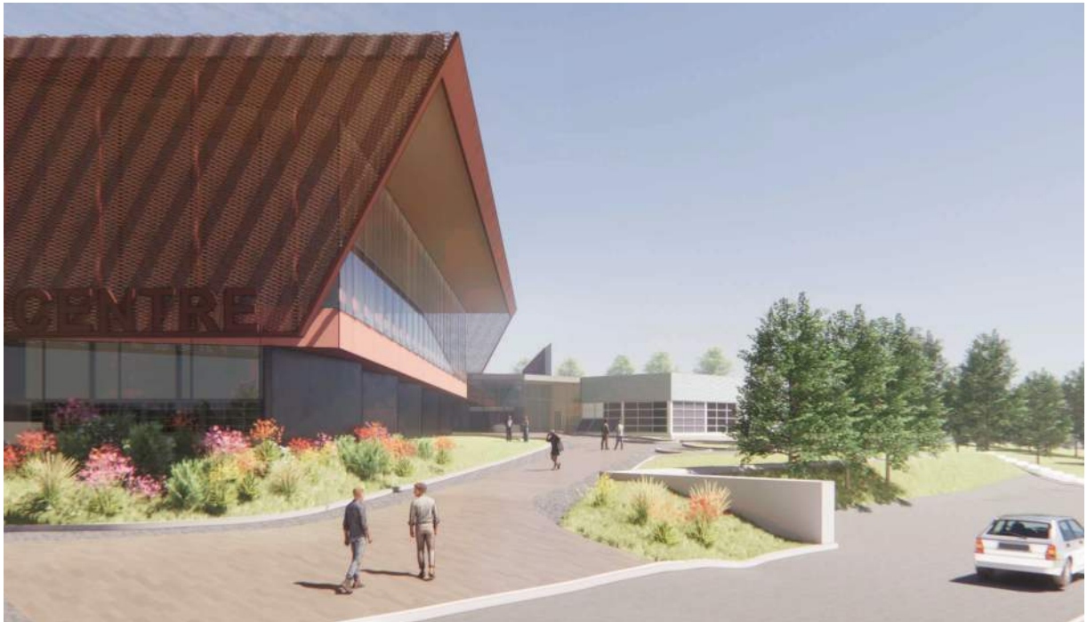
Building Exterior - South Entrance (Phase 2)
