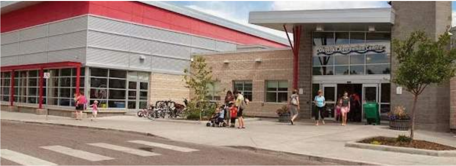
Image 1.1: Existing Facility Main Entrance
