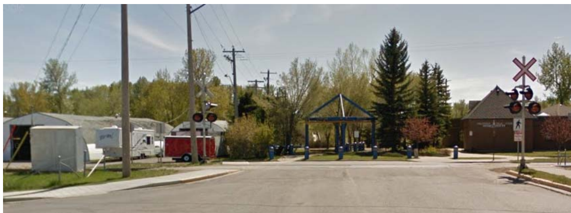
Figure 5.8 Signage and Signals, Southbound Veterans Way (Note orientation of signals to all approaches)
