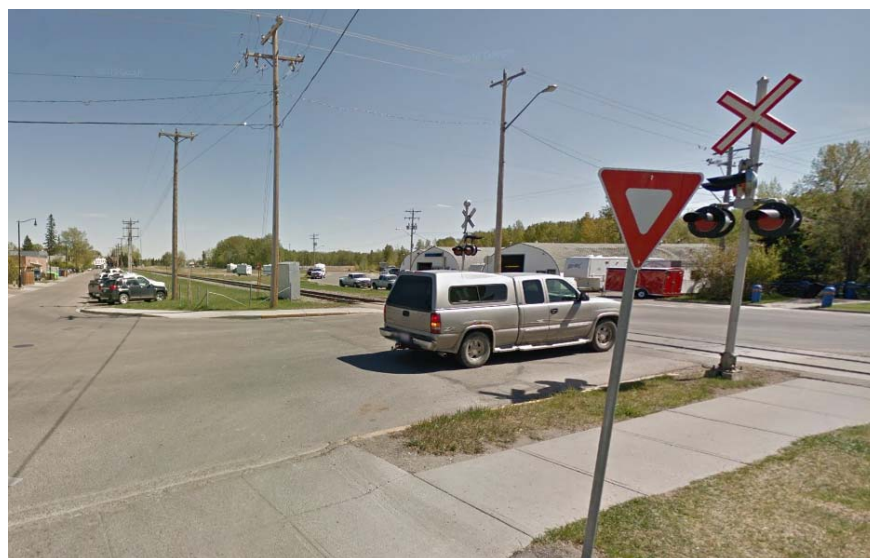
Figure 5.9 View of Rail Line and Signals, Eastbound Daggett Street
