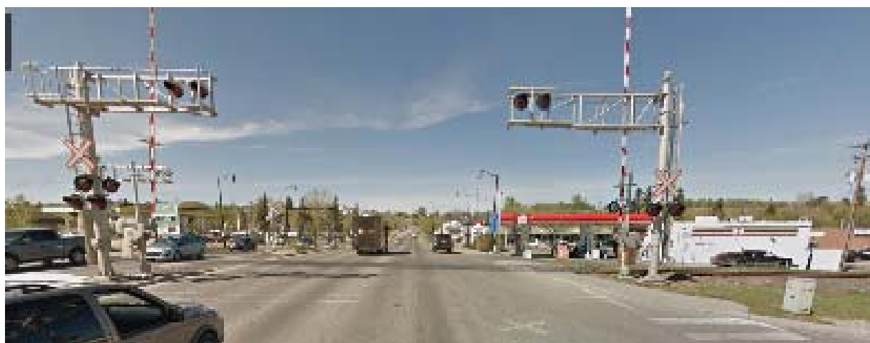
Figure 5.2 Gates and Signals, Northbound Northridge Drive Approach
