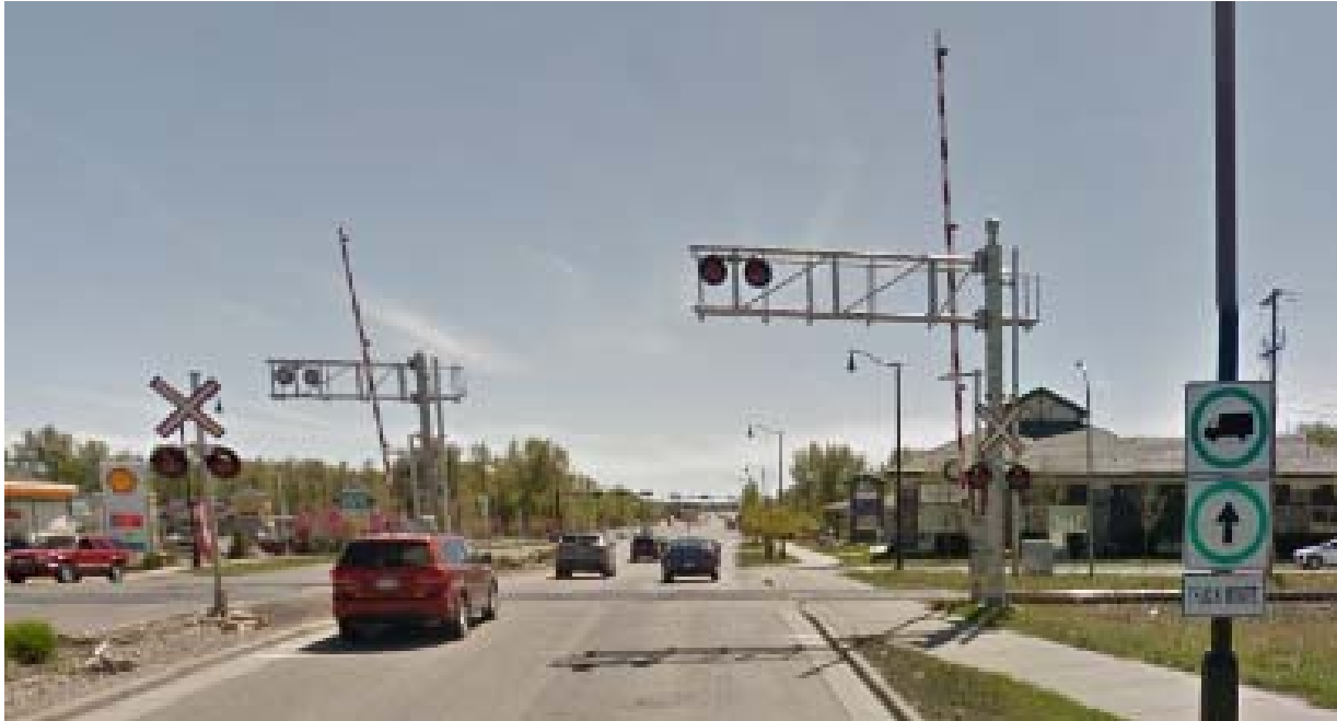
Figure 5.3 Gates and Signals, Southbound Northridge Drive Approach
