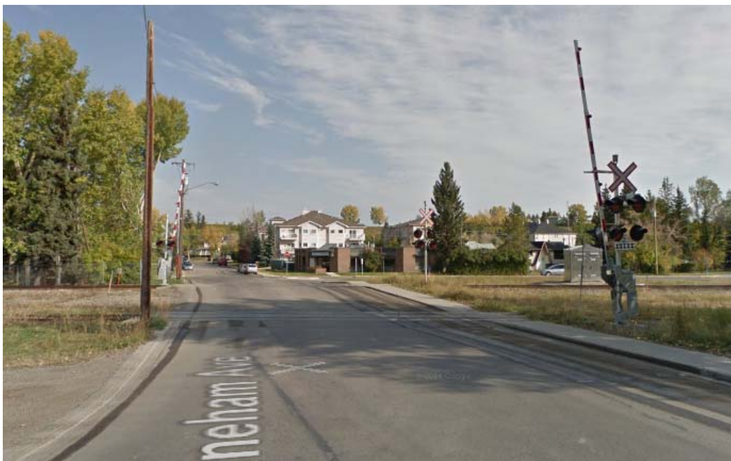
Figure 5.11 Gates, Signals, and Signage, Northbound Lineham Avenue (Note orientation of signals to northbound and to eastbound South Railway Street traffic)
