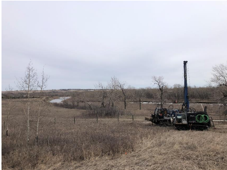
Photo 1: Geotechnical Drilling near Bow River
