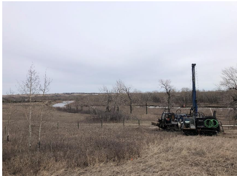
Photo 1: Geotechnical Drilling near Bow River
