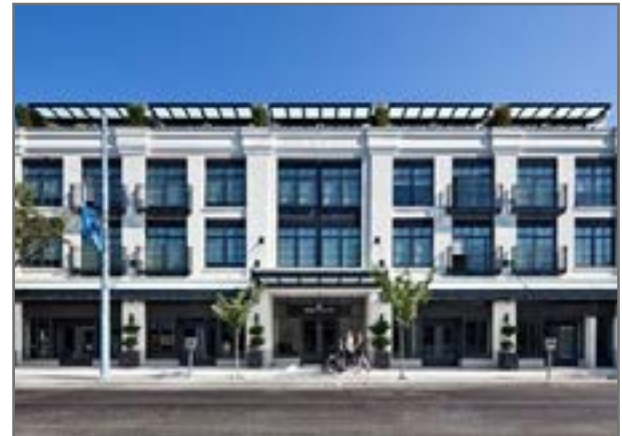
Retail, commercial, and business Uses should be integrated with residential for a Main Street feel
