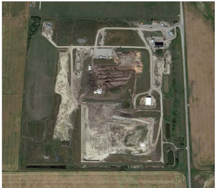
Figure 2: Aerial photo of Foothills Regional Landfill and Resource Recovery Centre
