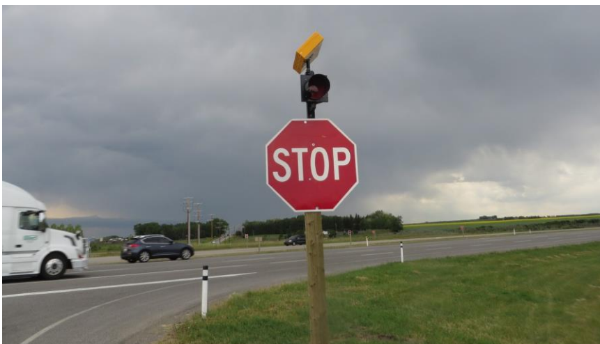
The Stop sign and flashing red light on the east approach.
