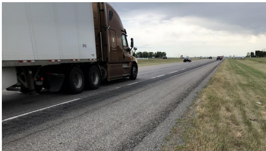
View of the start of the north approach right turn lane.
