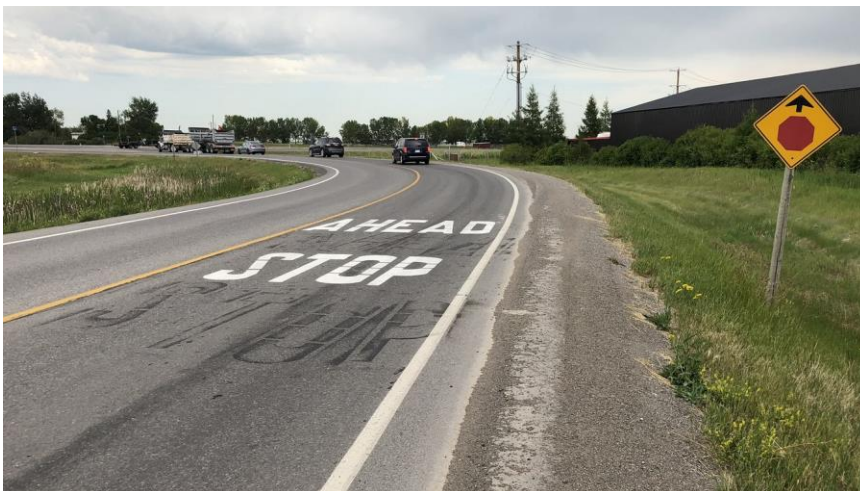
Looking toward the intersection from the Stop Ahead sign and word marking on the west approach.
