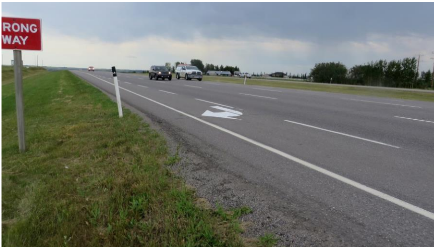
Looking south from the south approach right turn lane.
