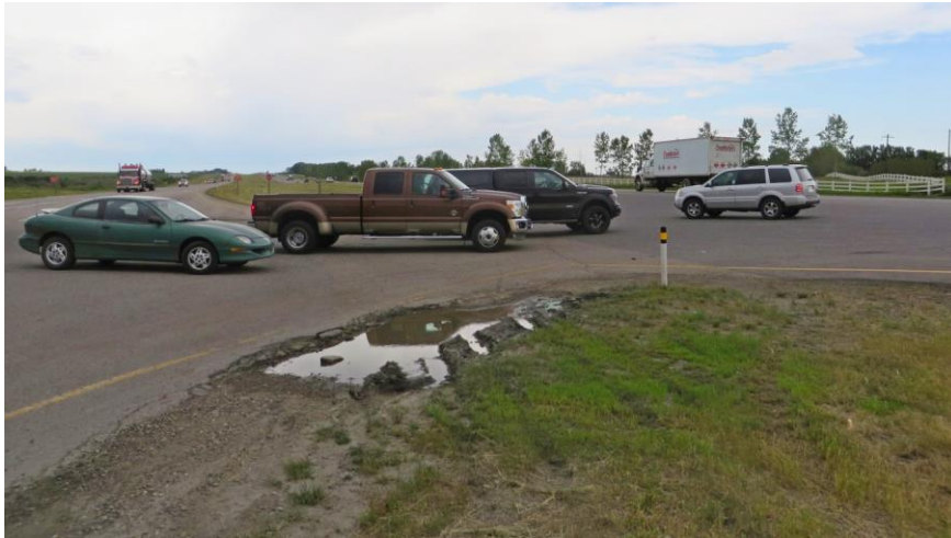
Looking north at the median opening.
