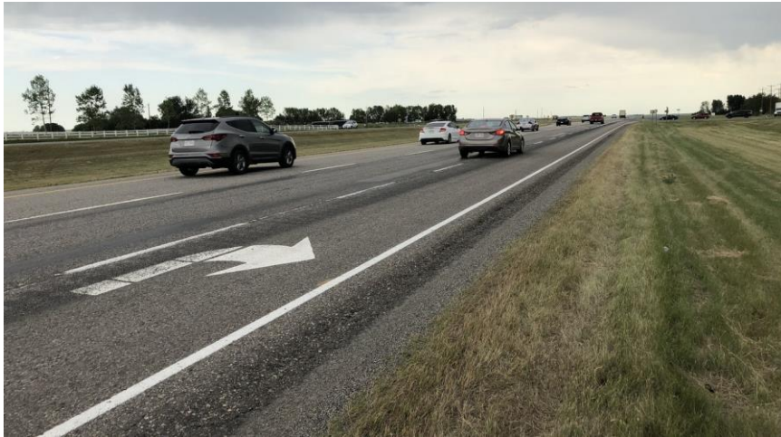
Looking toward the intersection from the north approach right turn lane.
