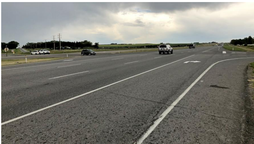
Looking toward the intersection from the south approach right turn lane.
