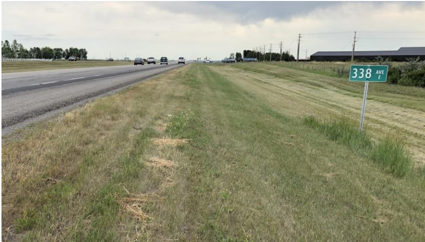
Advance Local Road Name sign on the north approach.
