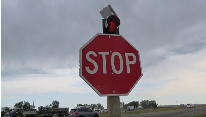
The Stop sign and flashing red light on the west approach.
