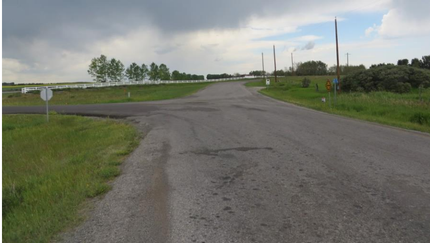
Looking north at the TR210 / RR291 intersection.
