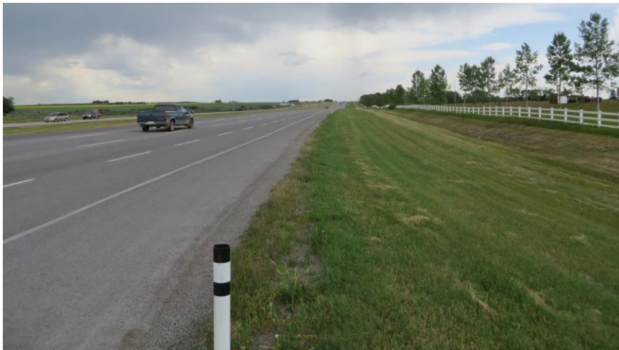
View to the north from the westbound right turn radius.
