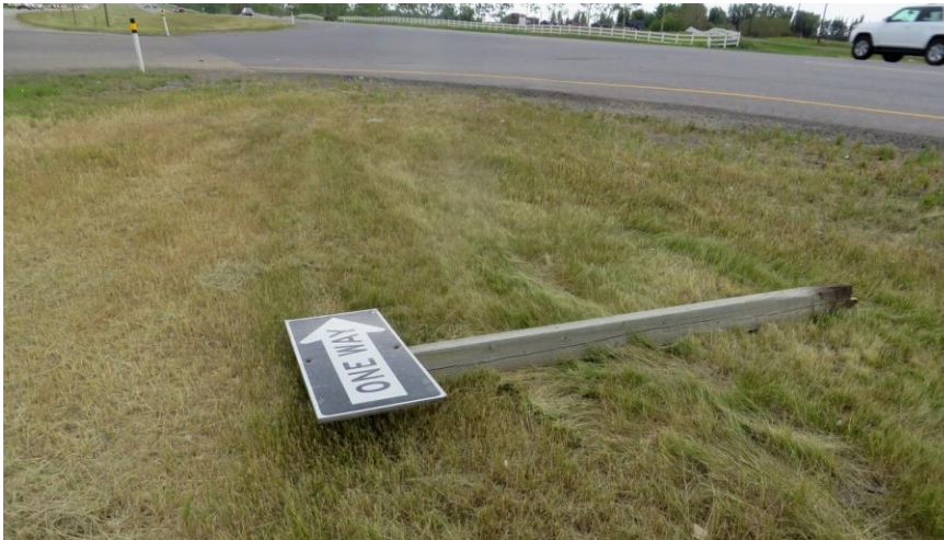
The One Way sign in the median beside the northbound left turn lane was knocked over.
