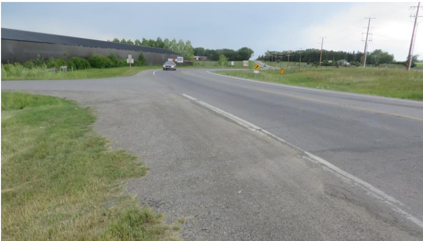
View west of the TR210 and 1064 th Drive E intersection.
