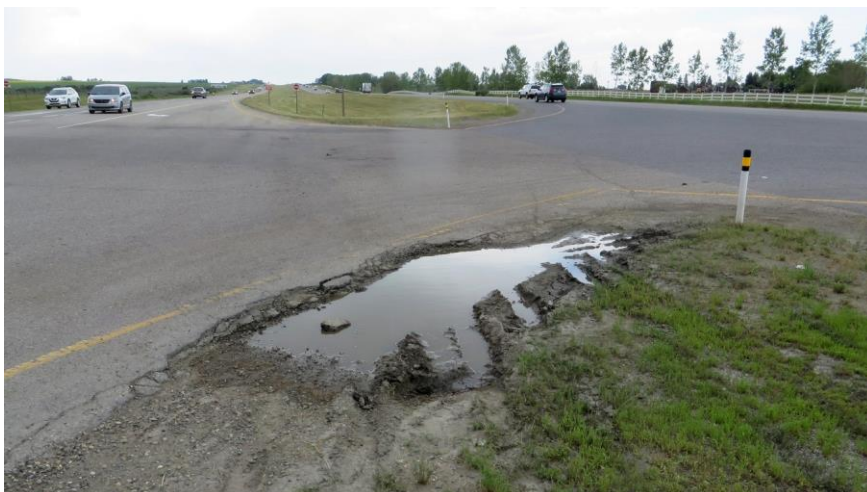
Looking north at the median opening.
