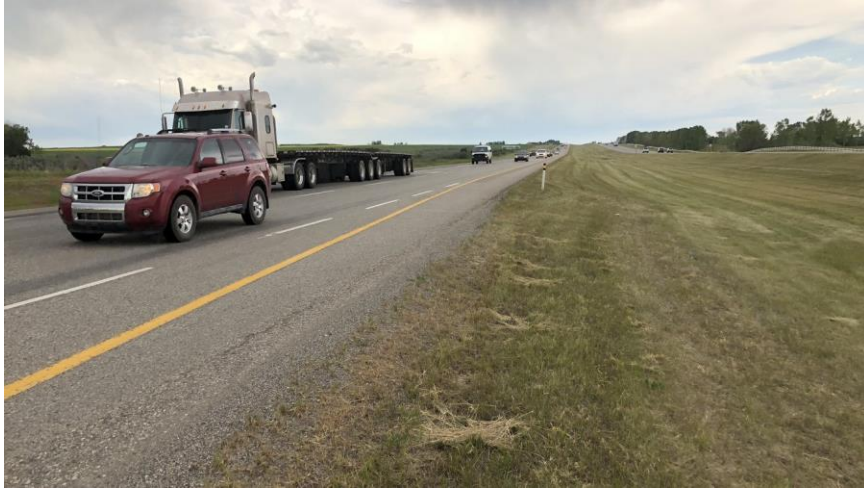
Looking north from the north approach left turn lane.
