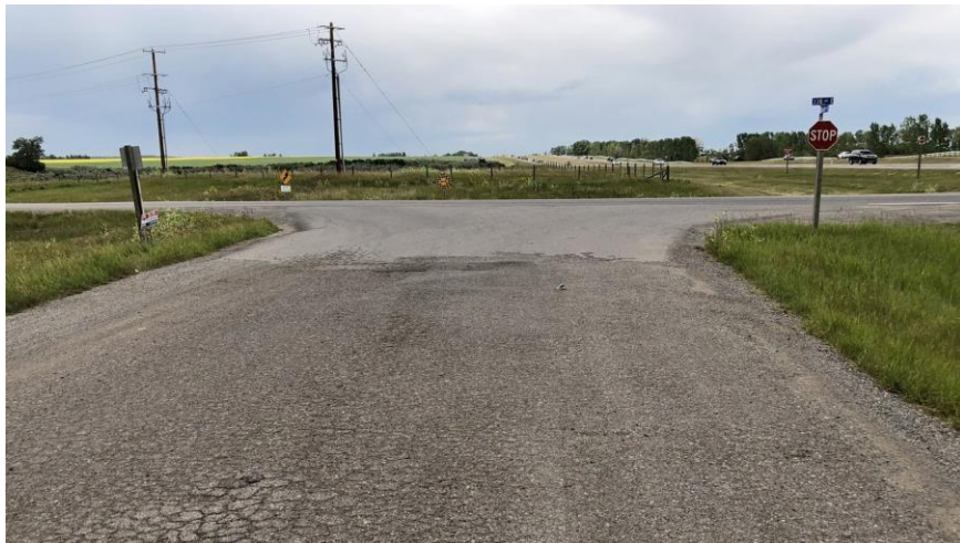
Looking north toward the TR210 / 1064 th Drive E intersection.
