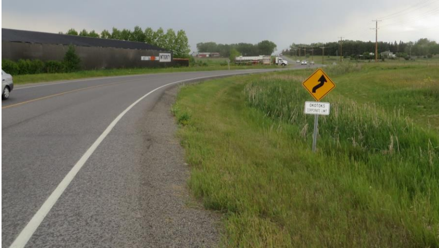
Looking west from the Reverse Curve sign on the west approach.
