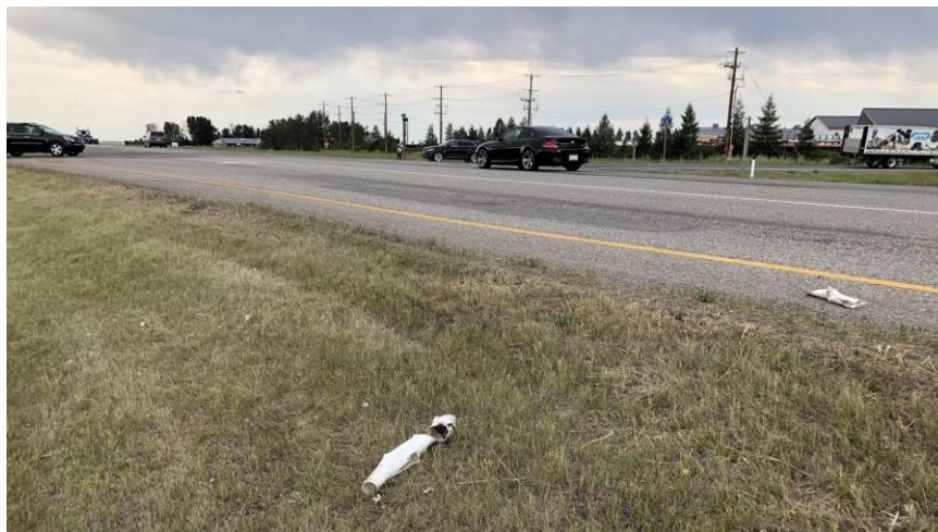
A delineator guide post beside the southbound left turn lane was knocked out of the ground.
