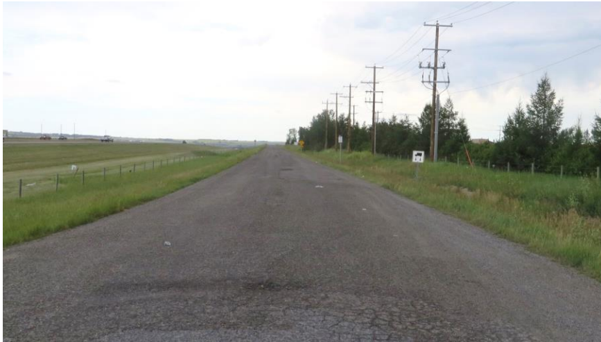
Looking south on 1064 th Drive E.
