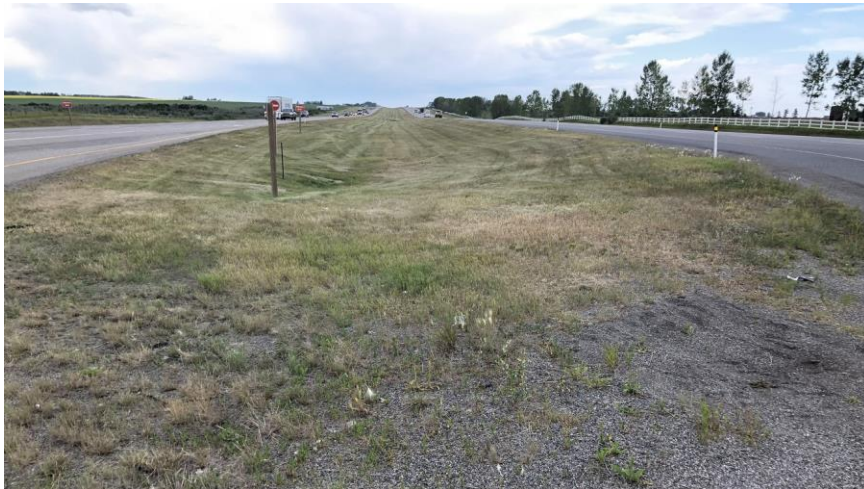
Looking north from the median opening.
