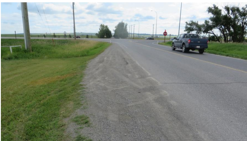
Looking towards the intersection from the west approach.
