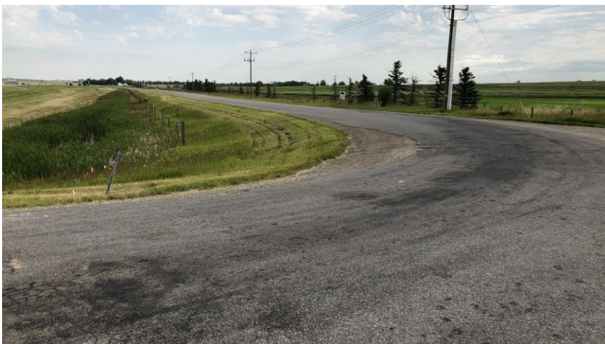
Looking north from the TR204/RR291 intersection.
