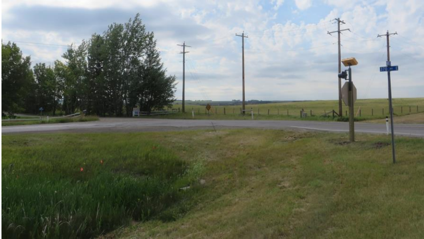
Looking toward the east approach from Highway 2.
