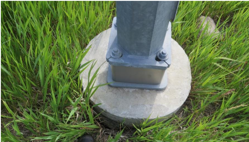
Street light pole base in southwest corner of intersection (Pole #17035312).
