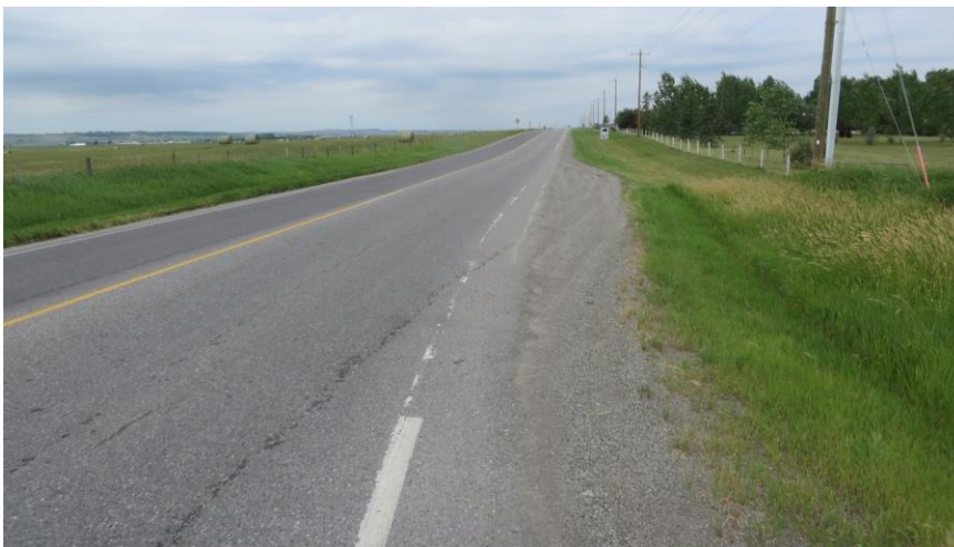
Looking west towards the west approach from intersection.
