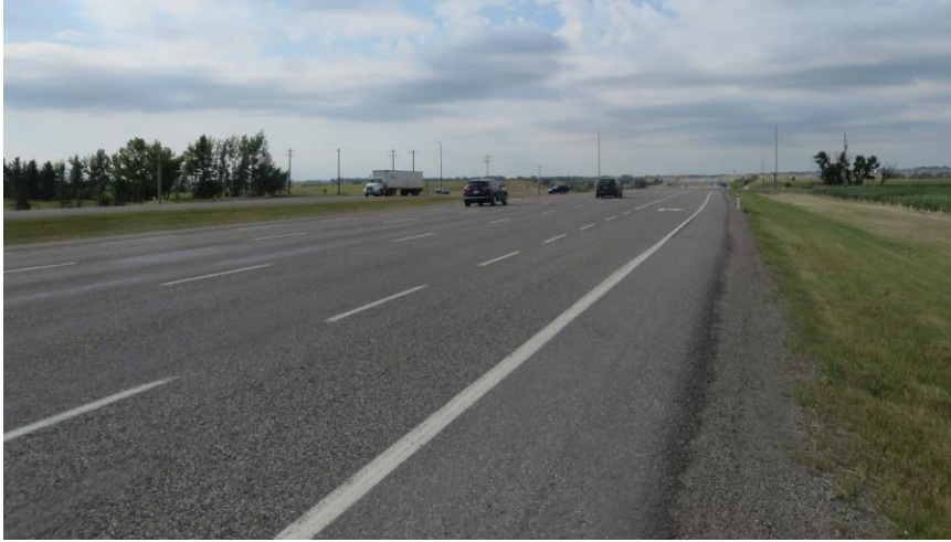
Looking toward the intersection from the north approach right turn lane.
