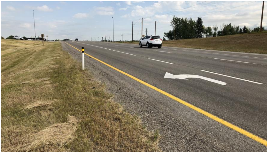
Looking toward the intersection from the south approach left turn lane.
