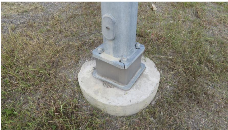
Street light pole base in south median (Pole #17035338).
