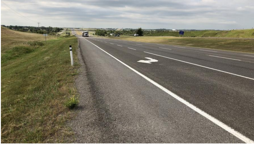
View of the south approach from the outside shoulder.
