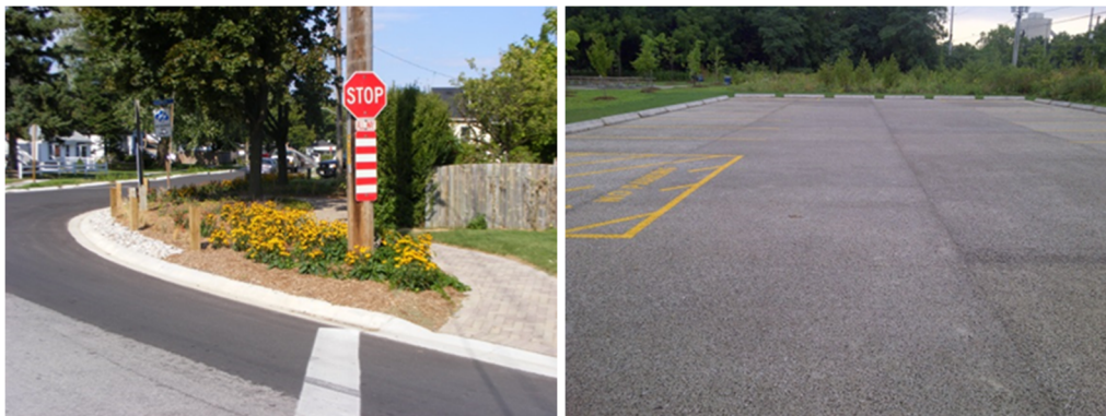
Figure 5.6- Source Control Retrofit within Parks, (From L to R) Permeable Pavement Parkette and Pervious Concrete Parking Lot (Source: Aquafor Beech Ltd.)
