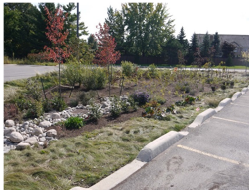
Figure 5.5 - Bioretention Source Control Retrofit at Portico Church (Source: Aquafor Beech Ltd.)
