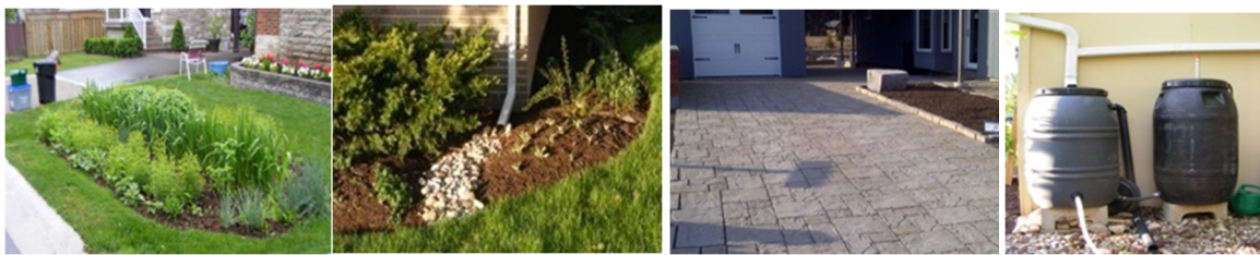
Figure 5.3 - Source Control Measures(From L to R) Bioretention, Downspout Disconnection, Permeable Pavement & RWH
