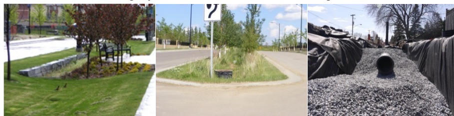
Figure 5.8 - Conveyance control measures.(From L to R): Vegetated Channel (Calgary), Bioretention/bioswale (Edmonton) and Perforated Pipe System (Mississauga)
