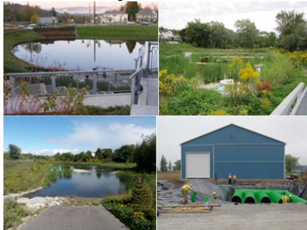
Figure 5.13 – End-of Pipe Controls (From L to R): Wet pond, Wetland, Hybrid and Sub-surface Facility (Source: Aquafor Beech Ltd.)
