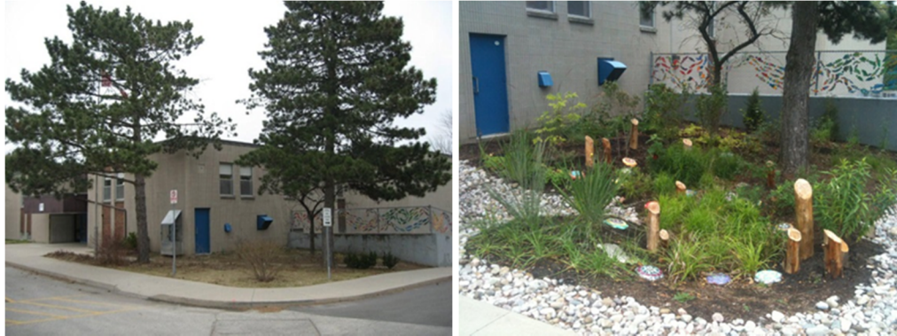
Figure 5.4 - Bioretention Source Control Retrofit at Green Glades Public School (From L to R) Before and After (Source: Aquafor Beech Ltd.)
