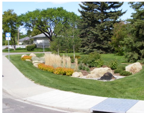
Figure 5.10 –Bioretention Retrofit of the Boulevard (Source: Aquafor Beech Ltd.)
