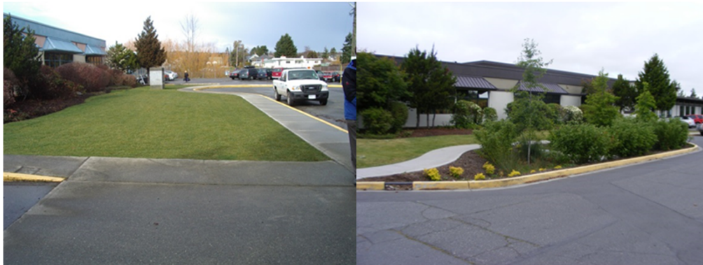
Figure 5.11 –Bioretention Bump-out Retrofit (L: Before (Source: City of Victoria), R: After (Source: Aquafor Beech Ltd.)
