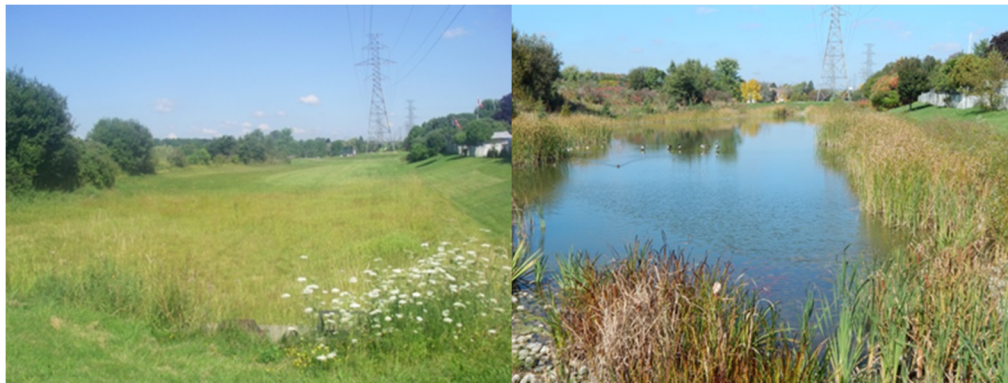
Figure 5.14 – Surface EOP Control Retrofit within the Drainage Network (From L to R): Before and After (Source: Aquafor Beech Ltd.)
