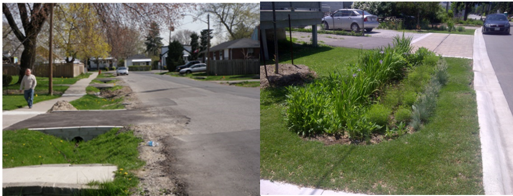
Figure 5.9—Bioswale Retrofit of an Existing Ditched ROW From L to R) Before and After (Source: Aquafor Beech Ltd.)
